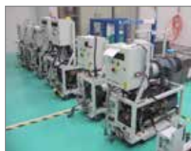
Pumped: Edwards in 3.5x exit
